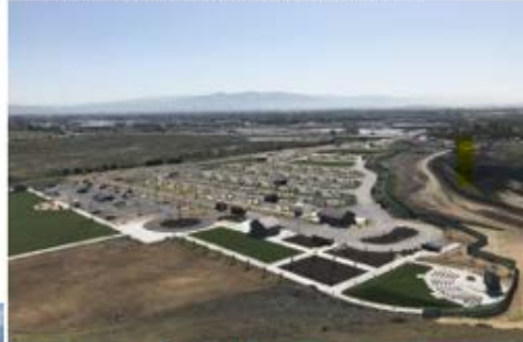
Dumbarton Quarry Campground, a month before the Grand Opening
